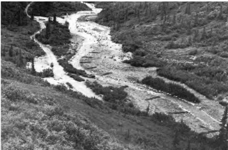
Brush bars for floodplain stabilization may be seen on either side of the channel in this aerial view of the lower half of the 1991 study reach on Glen Creek in Denali NP.
