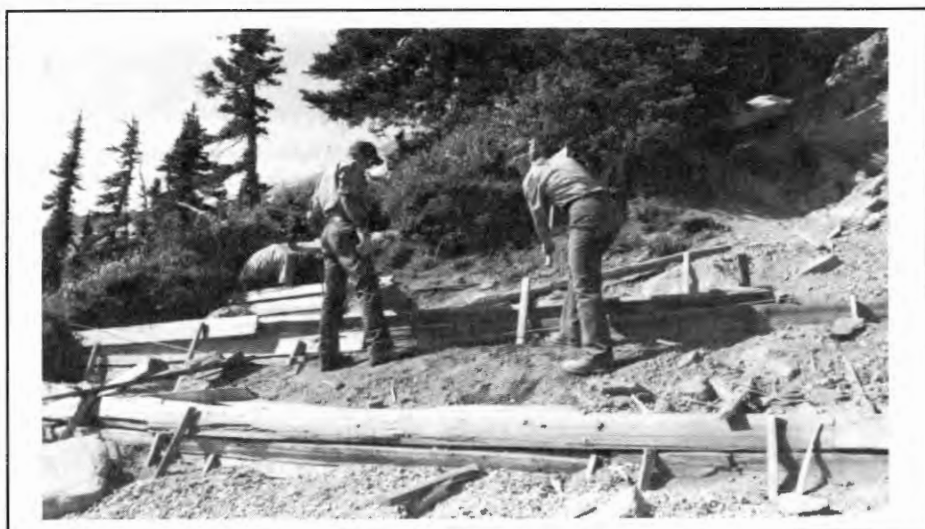
Restoration crew is shown here installing stabilization bars or silt dams; the area in the foreground has been filled with gravel and will next be filled with soil.
