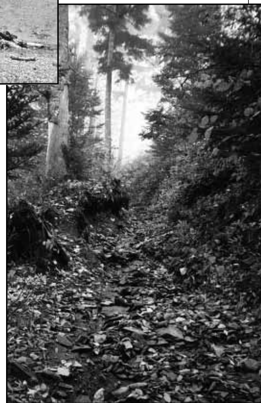
Figure 3. Trails within Great Smoky Mountains National Park are degrading. Not only is visitor safety a concern, but soil is eroding into streams, threatening aquatic life, and vegetation is being trampled. The new construction evaluation process considered these multiple impacts and funded the project, which will repair, rebuild, realign, or relocate 400 miles of trail.
