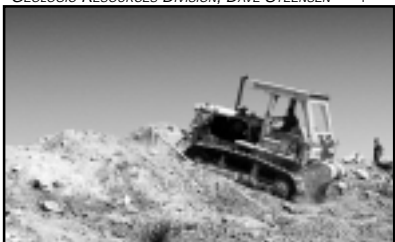
An Army Reserve bulldozer recontours the sandstone quarry at El Malpais National Monument
