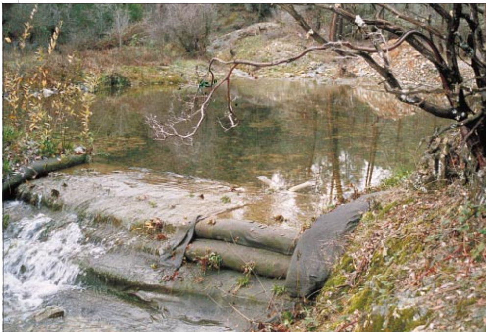
Fig. 4. A sediment pond was constructed within the lower reaches of the watershed to monitor erosion before and after restoration work. After three years, it will be removed and the stream restored to its natural course.
