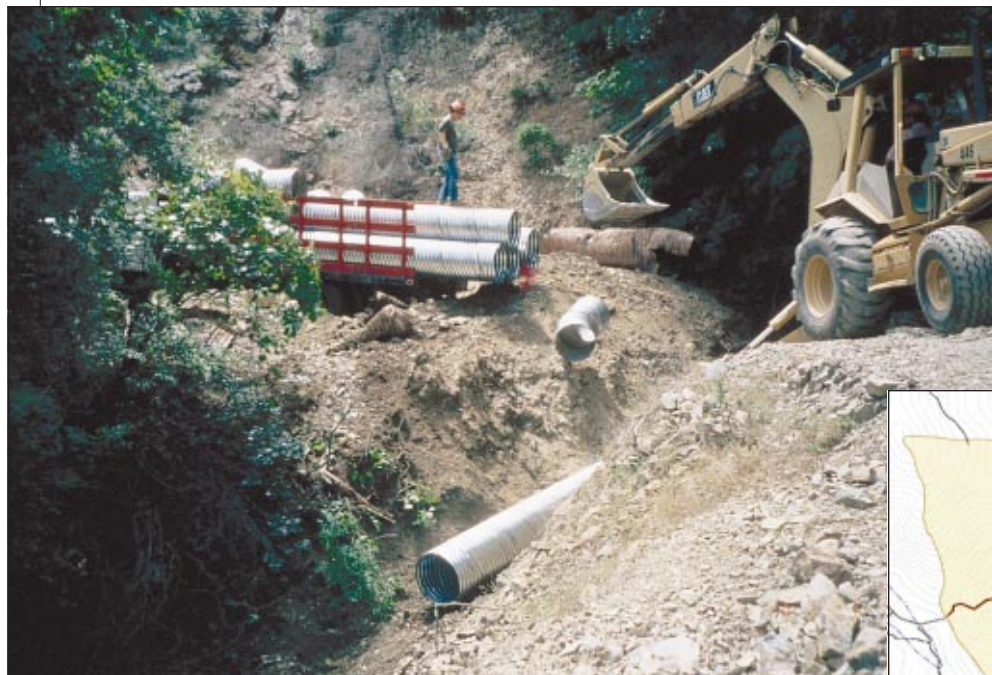
Fig. 2 (left). Heavy equipment is used to treat the drainage problems posed by the old logging roads. Here, a culvert is installed to restore natural drainage patterns and reduce erosion of the fill.
