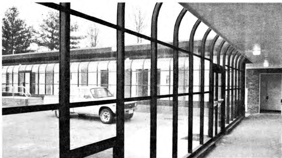
A passive solar walkway connects all offices and laboratories with the administrative area, conference room and common use area of the Center for Urban Ecology. The brick columns define the former vehicle bays. This modification of the former Palisades maintenance yard allows total utilization of existing space for laboratory and office purposes, rather than sacrificing any to interior passageways.
