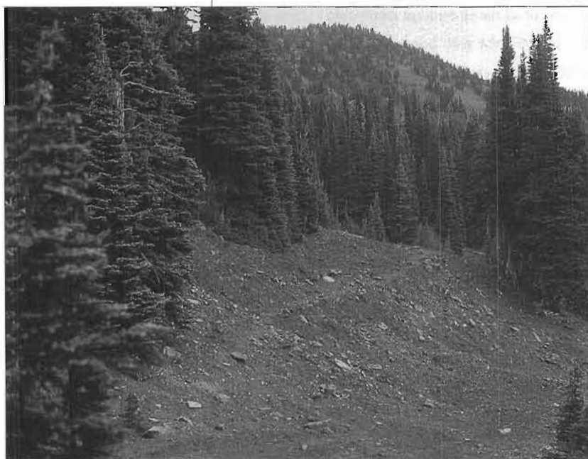
Army National Guard and Reserve engineering units restored an abandoned road and an unused portion of a campground at Mount Rainier National Park (Washington) during 1997. The process involved removing the oiled road surface (top), returning soils to their original horizons (middle), and reestablishing the original contour (above), creating the best conditions for revegetation.
