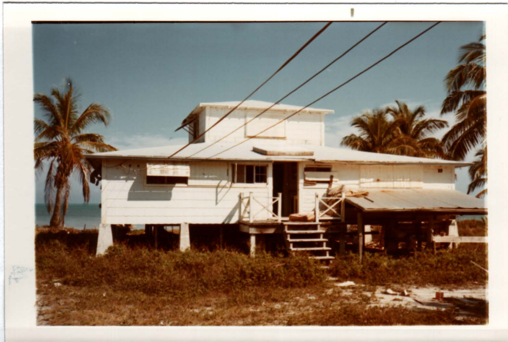
BUILDING NO. ONE
