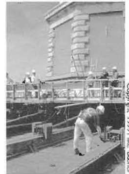
Moving the 4,800-ton lighthouse was no small engineering feat. Contractors employed 100 jacks to keep the lighthouse level while five hydraulic rams gently nudged it along iron beams lubricated with soap to its new resting place 2,900 feet away. The operation went smoothly, taking 23 days and causing no damage to the 130-year-old treasure.
