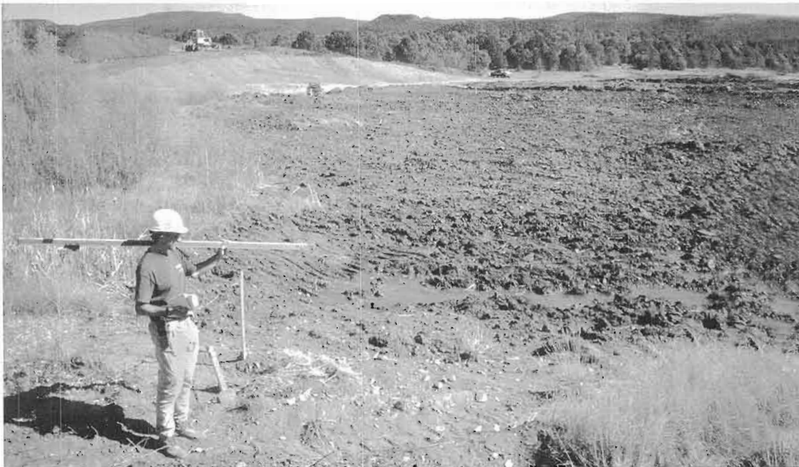
Most earthmoving contractors are experienced in creating smooth surfaces needed for roads or parking lots, but may not know how to interpret the degree of undulation or "roughness" called for in wetland projects. For the Glorieta Creek rehabilitation project, a member of the design team was on-site at all times during the earthmoving phase, interpreting these details for the contractor and checking elevations with a laser level.
