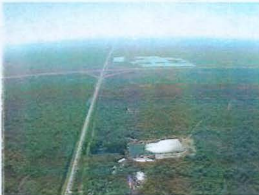
Photo 2-5. Aerial view of Interstate 75, looking south.
