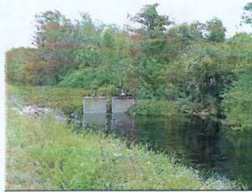
Photo 2-8. Photo of water flowing over the crest of Gate 6B.
