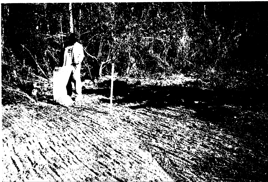
P. #58 Test Pit #11. Backfilled area and final hand clean up.
