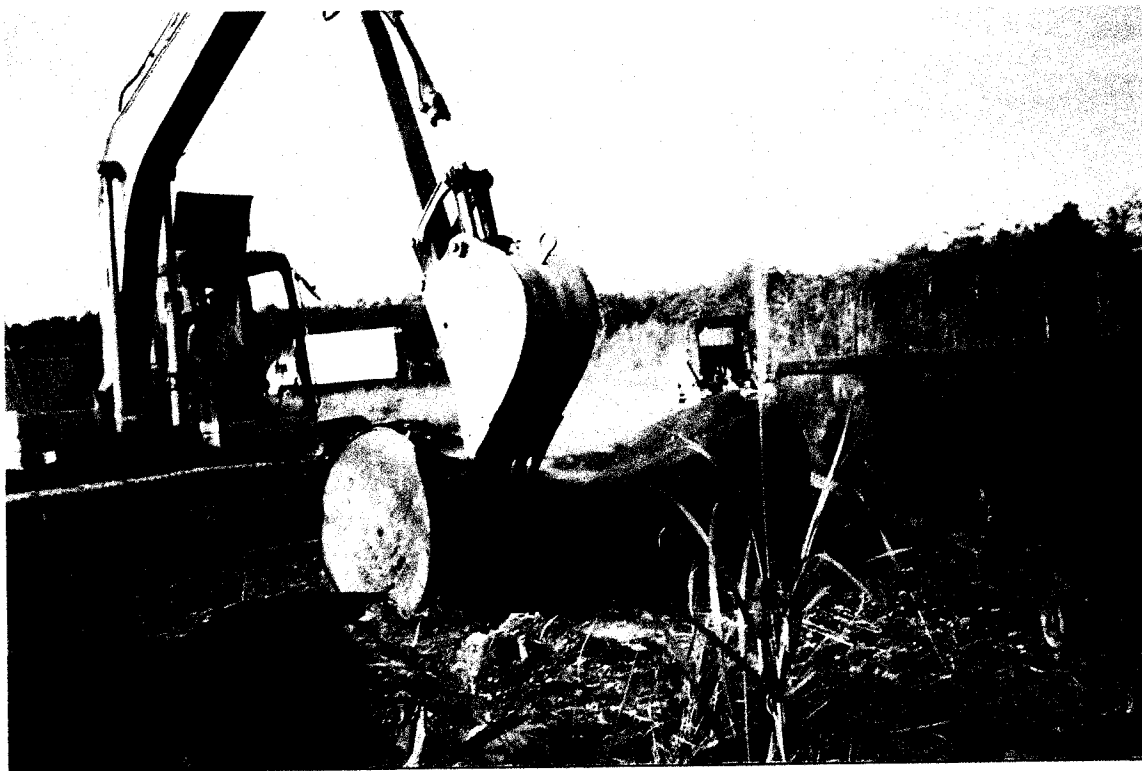
P. #20 Crushing empty, rusted tank. Test Pit #1.
