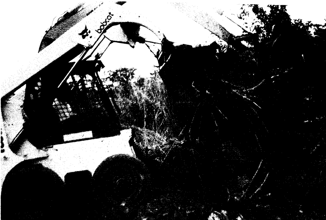
P. #75 Removing surface debris with Bobcat assisted by track excavator.
