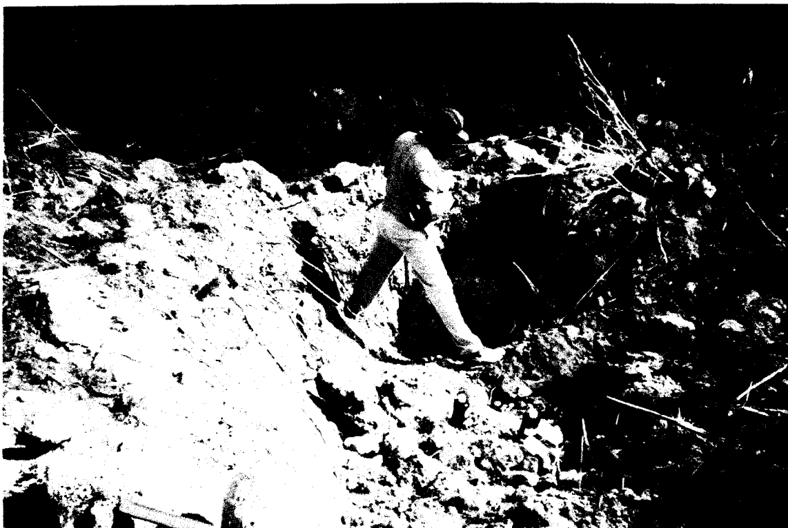
P. #19 Test Pit #1. Taking soil samples.
