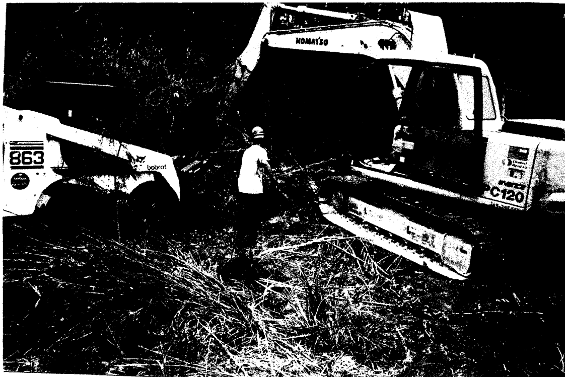
P. #16 Test Pit #1. Removing debris from the area.
