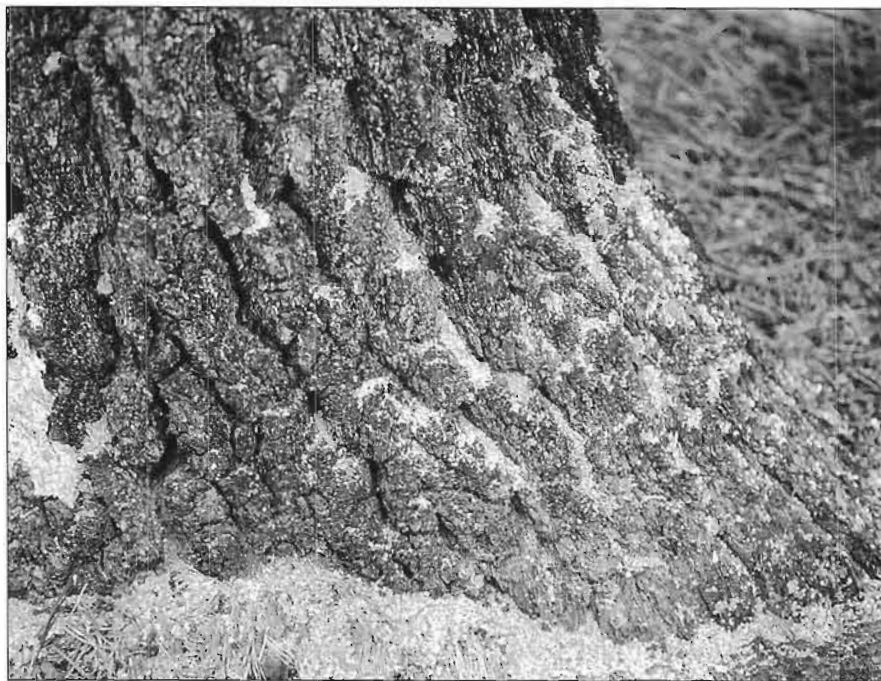
Reddish-brown boring dust around base of tree
