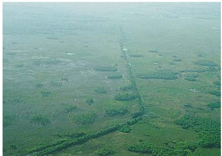
Photograph 2. Shot looking southwest at the bend in the southern irrigation canal. The berm switches sides at the bend.
