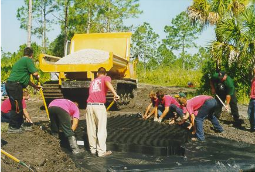
ORV trail test area. Crew installing Geoweb over Geotextile matting, one of the methods investigated in strengthening ORV trails in high traffic trail areas.
