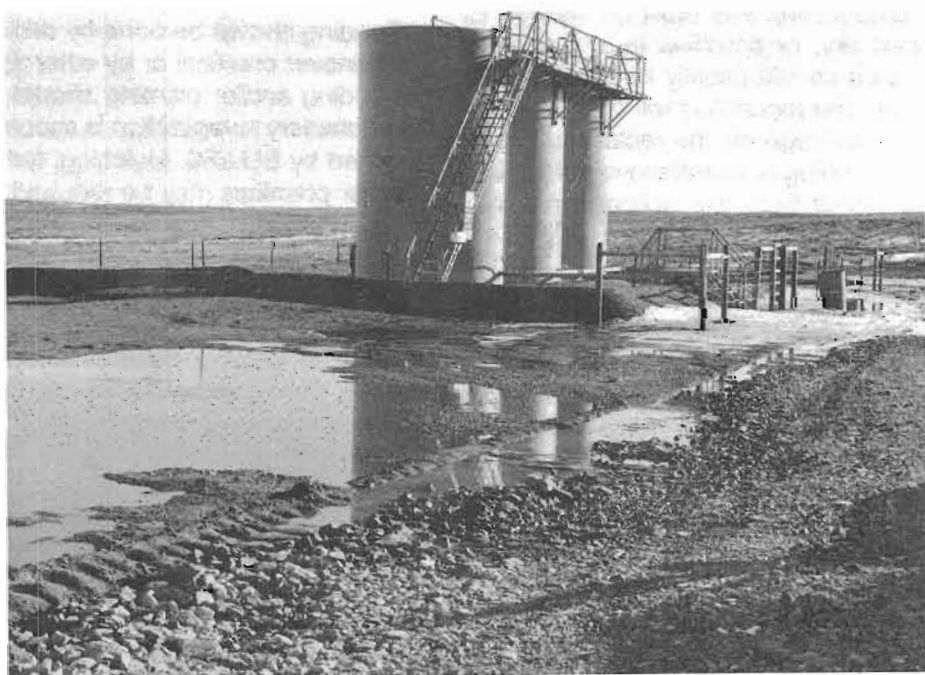
PHOTOGRAPH 5. TYPICAL PRODUCTION FACILITY FIREWALL
