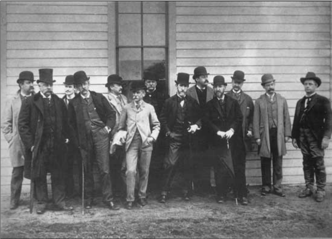
Fig. 3 Although no photograph of the Senate Park Commission members together is known to exist, this 1892 view of architects and officials of the World's Columbian Exposition shown Daniel H. Burnham, far left; Charles F. McKim, third from right; and Augustus Saint Gaudens, sixth from right (with top hat). The fourth member, Frederick Law Olmsted, Jr., was an undergraduate student at Harvard at the time, George Browne Post, president of the AIA in 1896-97 and an important figure in the planning of the 1900 AIA Annual Meeting, is second from the left. Chicago Tribune , 26 January 1930. Photograph courtesy the American Institute of Architects Library and Archives.
