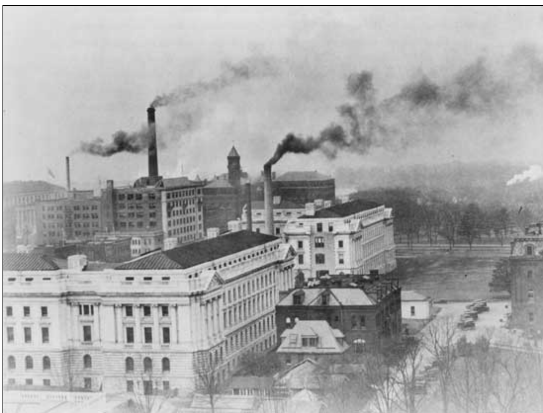
Fig. 6 In the days when soft coal was the primary fuel for heating and power plants, both smoke and smokestacks marred the views from the Mall. This photograph shows the effect on the wings of the new Agriculture Building, before the center section was erected and the old buildings demolished. The Commission of Fine Arts, during the January 1916 meeting, objected strongly to the proposed construction of a central heating plant at 14th Street and the Washington Channel, roughly the area in the left background of this photograph. It was to have had four stacks, each 16 feet in diameter and 188 feet high. The commission noted the effect of both the smoke and the stacks from the Mall, the Lincoln Memorial and other new Mall buildings, the Washington Monument, and the White House. The heating plant was not built. Undated photograph, ca. 1920. Commission of Fine Arts
