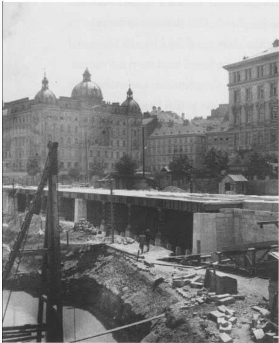
Vienna: Donau Kanal; work on quay and subway
