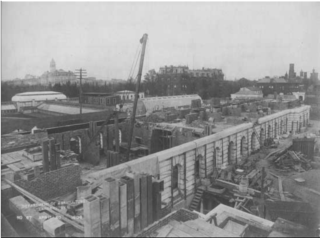
Fig. 12 Construction of west wing of the Department of Agriculture building, April 1906. Shows brick bearing wall construction and extensive tile flue system for ventilation of laboratories. View is to the northeast, with Conservatory and old Post Office building at top left, old Department building at top center, and Smithsonian castle at top right. Author's collection.
