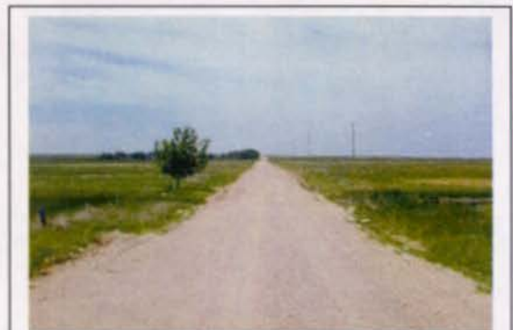
12. View of Road W facing west from southeast corner of property.
