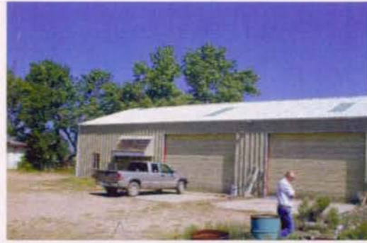
2. Metal maintenance shed located to the east of the ranch house (see previous).
