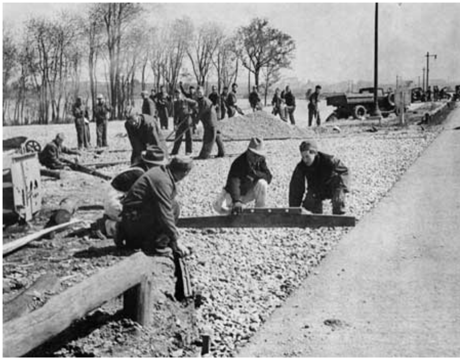
CCC Construction of Parking Area at Roaches Run
