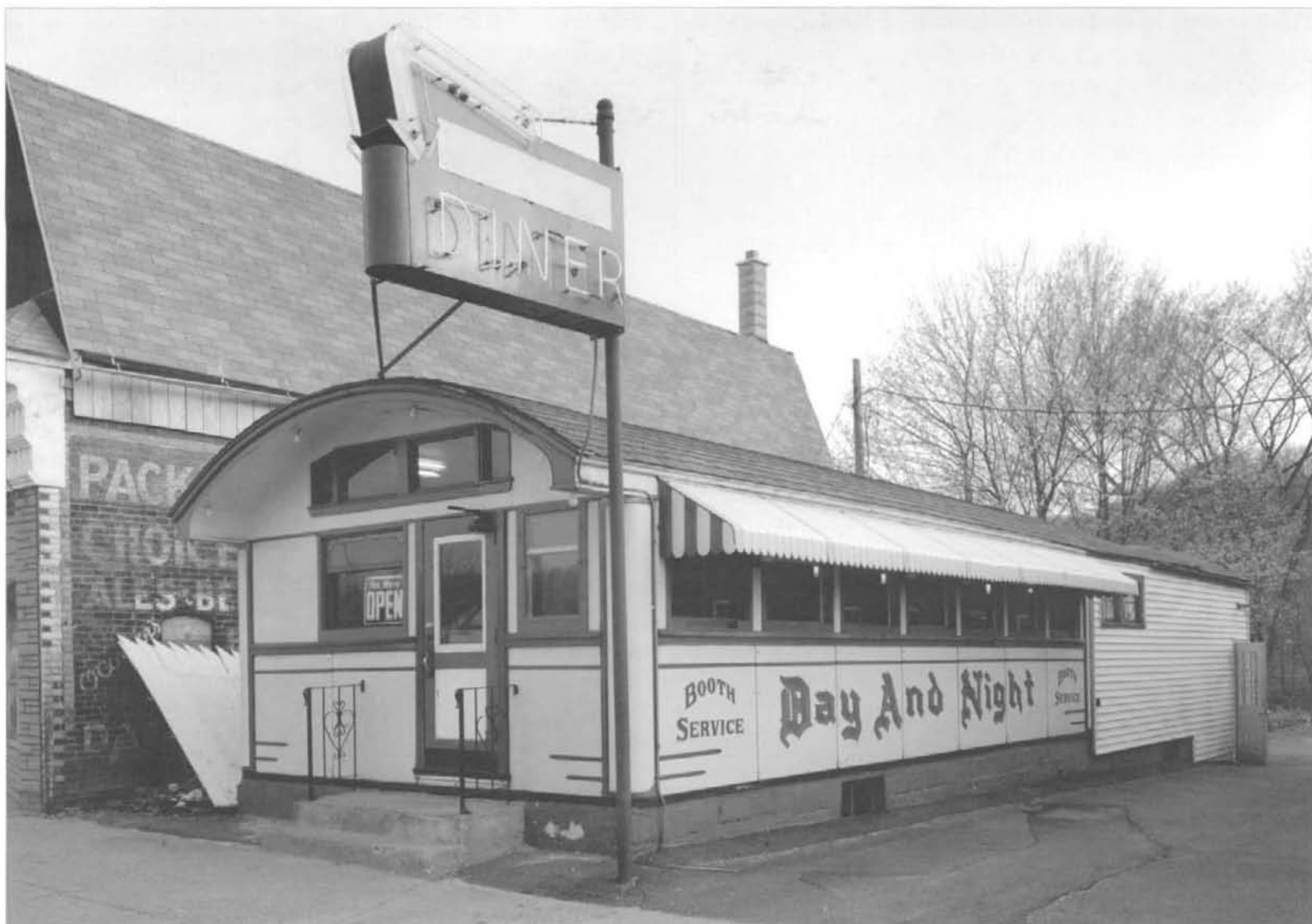
Day-And-Night Diner , 456 North Main Street, Palmer, Massachusetts; Jack E. Boucher, photographer, 1987; HABS No. MA-1231. The Day-And-Night is a wonderfully intact example of the Worcester Lunch Car. Built in 1923, the diner is constructed of sheet metal and its exterior enameled in cream with red details. It was recorded as part of a statewide HABS survey sponsored by the Massachusetts Historical Commission.
