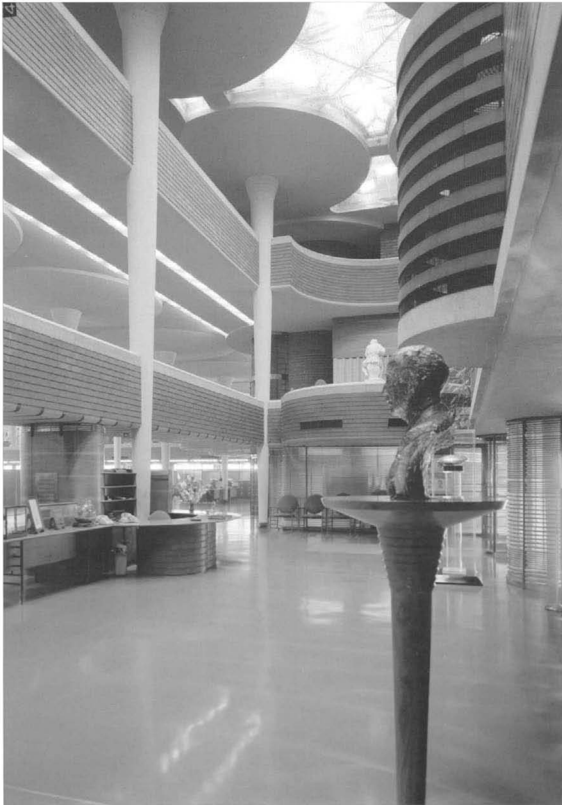
Johnson Wax Corporation Building , 1525 Howe Street, Racine, Wisconsin; Jack E. Boucher, photographer; HABS No. WS-284. The Johnson Wax building is one of the best known designs of famed architect Frank Lloyd Wright. Built between 1936 and 1939, it is noted for its open space, cantilevered balconies, glass-tube ribbon windows, and unusual lily-pad columns.
