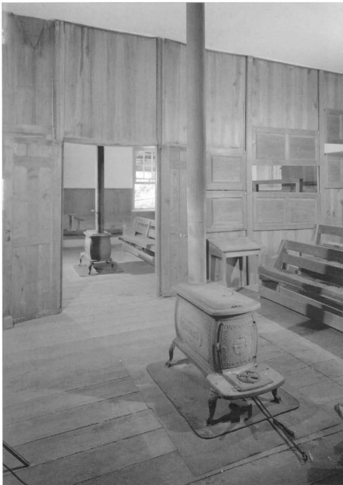
Bradford-Marshallton Friends Meeting House, Marshallton, Pennsylvania; Jack E. Boucher, photographer, 1999; HABS No. PA-1105. The meeting house was built in 1759 and is still in use, although without central heat or electricity. It was divided by partitions into identical apartments for men and women, as aptly demonstrated by this photograph. Its documentation was part of a study of the Friends meeting houses of the Delaware Valley.
