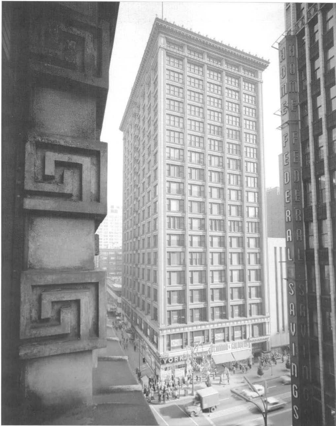
The Republic Building , 209 S. State Street, Chicago, Illinois; Richard Nickel, photographer, 1960; HABS No. IL-1004. This early skyscraper was designed by Holabird & Roche and built in 1905 on Chicago's Loop. It included fireproof, steel frame and terra cotta construction. The documentation was donated by Skidmore, Owings, and Merrill, and was undertaken prior to the building's demolition in 1961.
