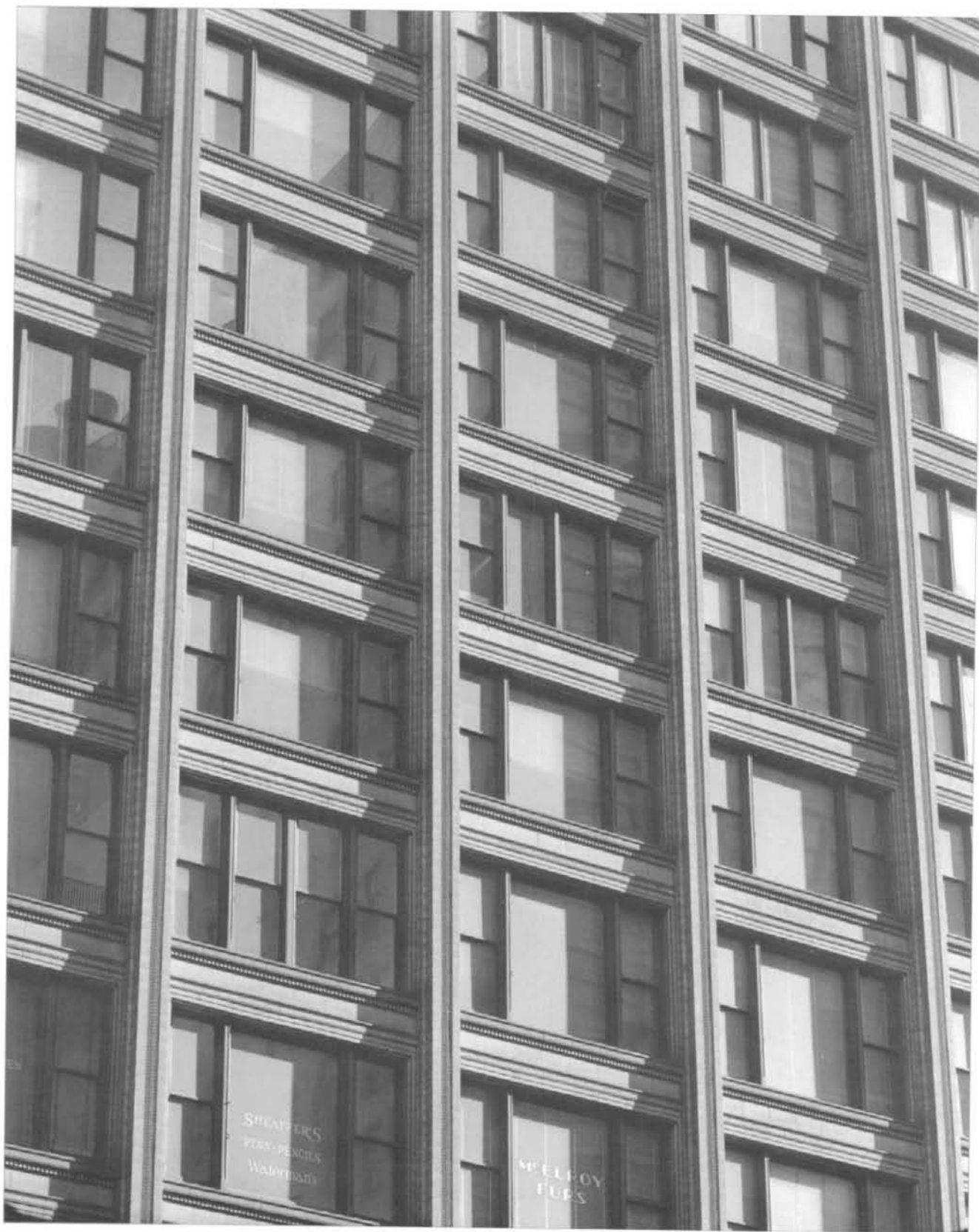
Detail, Republic Building. The three-part window seen here—consisting of a large, fixed central panel flanked by smaller double-hung sash windows—came to be known as the “Chicago Window.” It was used in many of the city’s landmark, early twentieth century skyscrapers.
