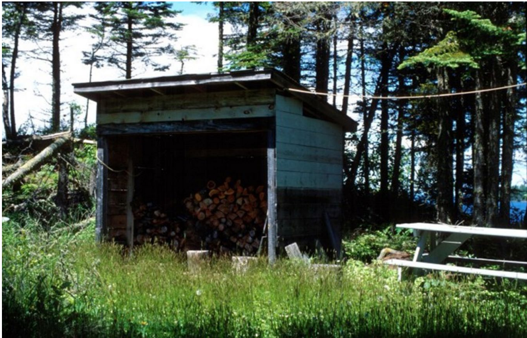
Barnum woodshed, facing northeast. (Diane Cook/NPS 2000)
