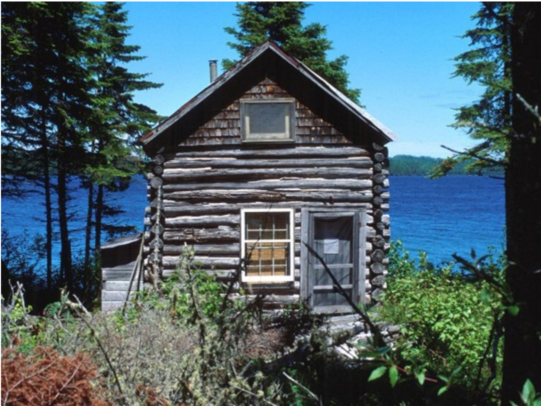
Johns Log Cabin, facing north. (Diane Cook/NPS 2000)
