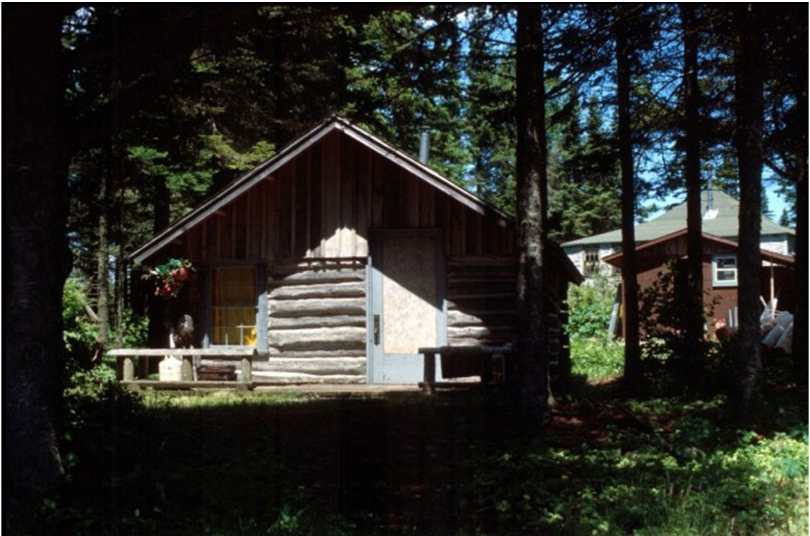
Andrew's Small Log Cabin, or Barnum Cabin, reconstructed. (Diane Cook/NPS 2000)
