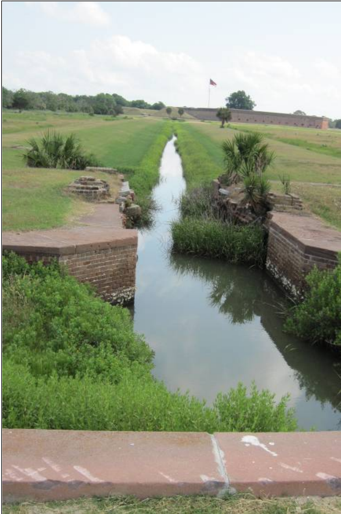
Figure 3. Example of drainage canal at Fort Pulaski National Monument.
