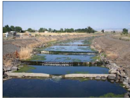
Mill Creek near the city of Walla Walla. Note the flood control structures and shallow channel, both of which contribute to increased water temperature.
