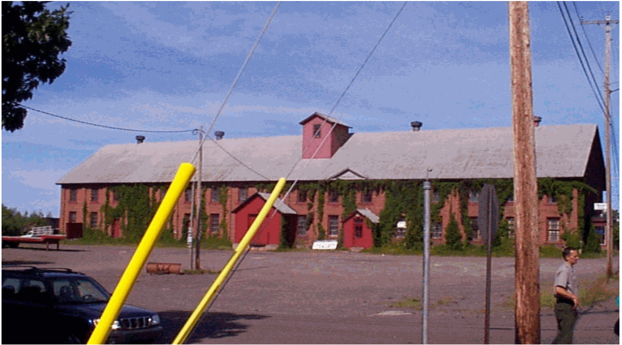
C&H Warehouse Number One Cultural Landscape
