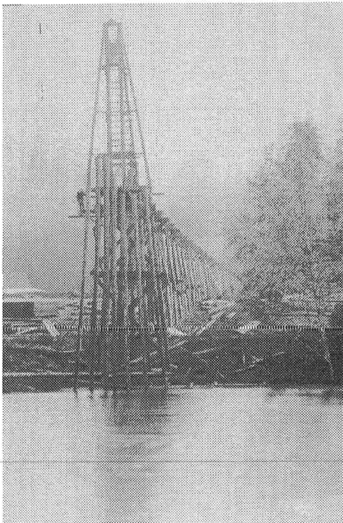
Piling approach to the second crossing of the Sol Duc #3690
