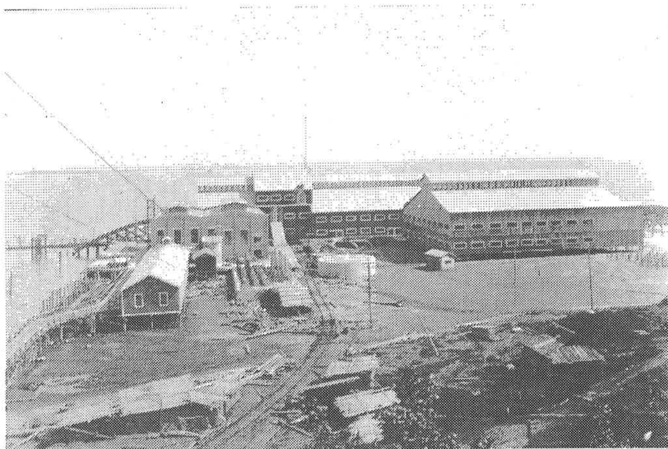
Mill in Port Angeles under construction #38030
