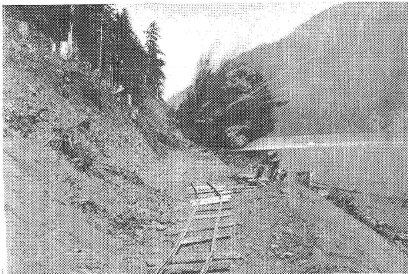
Blasting on the north side of Crescent Lake, with construction track to remove material. No Curtis number; Album 164A pg. 30.
