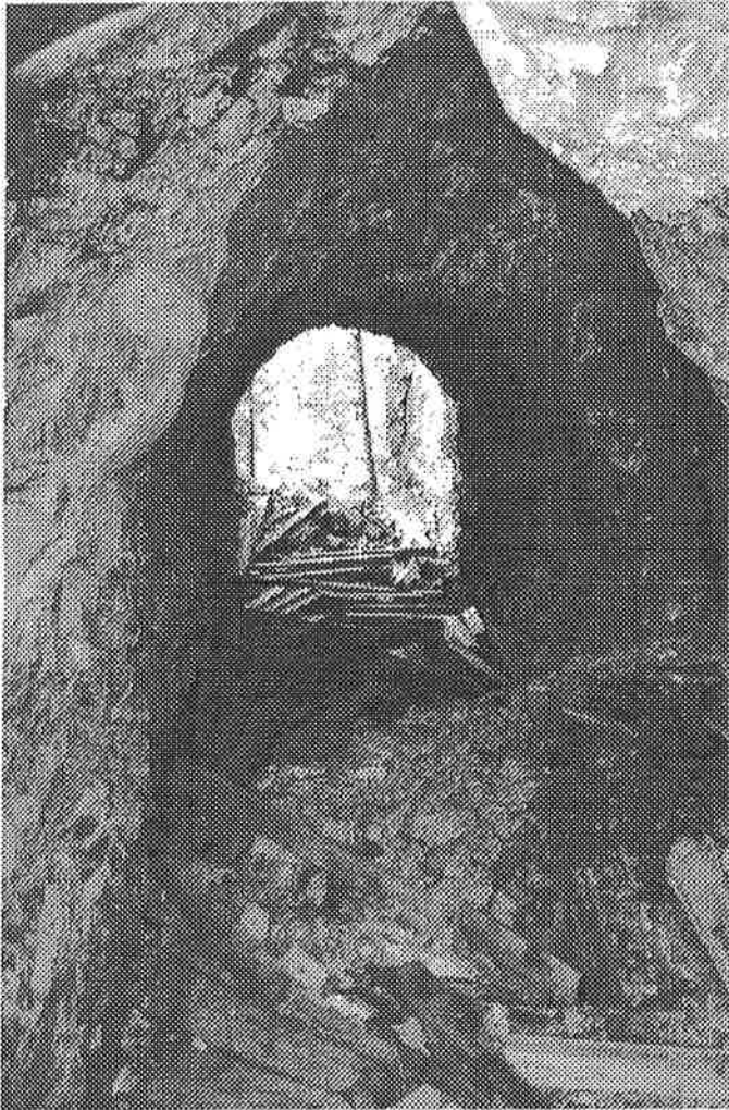
Photo D1-15 View through tunnel 2, segment 8
