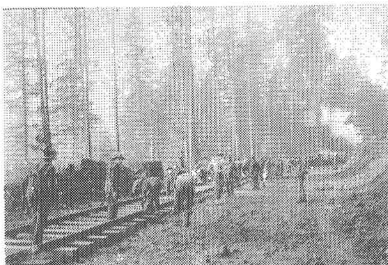
SPD steel gang spiking down the rails #36913
