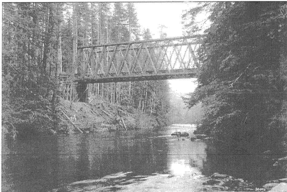
View of first Sol Duc bridge #38072
