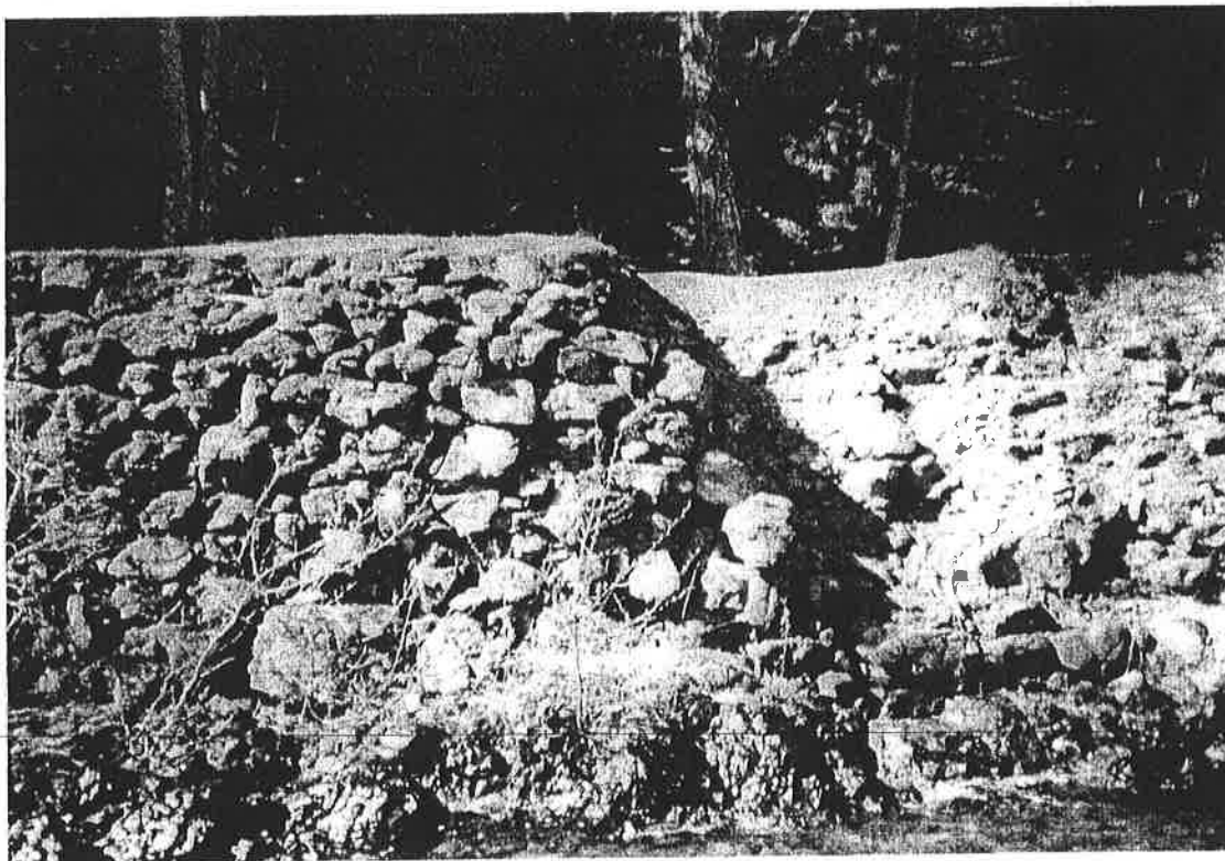
NPS2 Revetment with facing stone, segment 9
