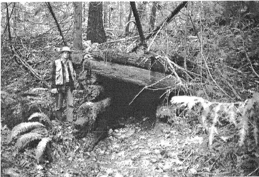
Photo W1-3 Culvert on segment 9
