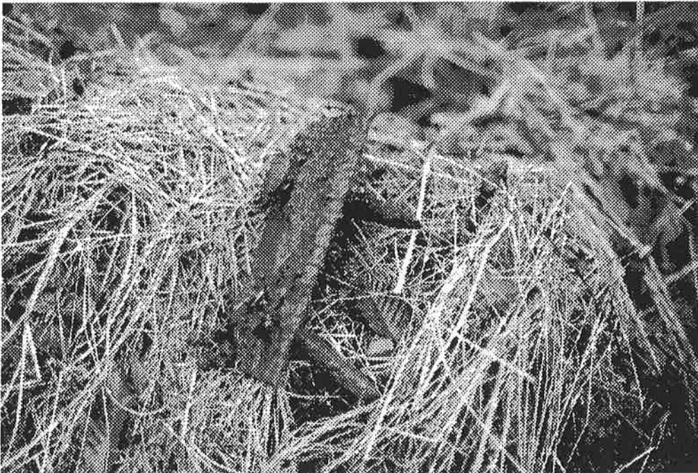
L2-8 Tie plate with spikes on segment 11
