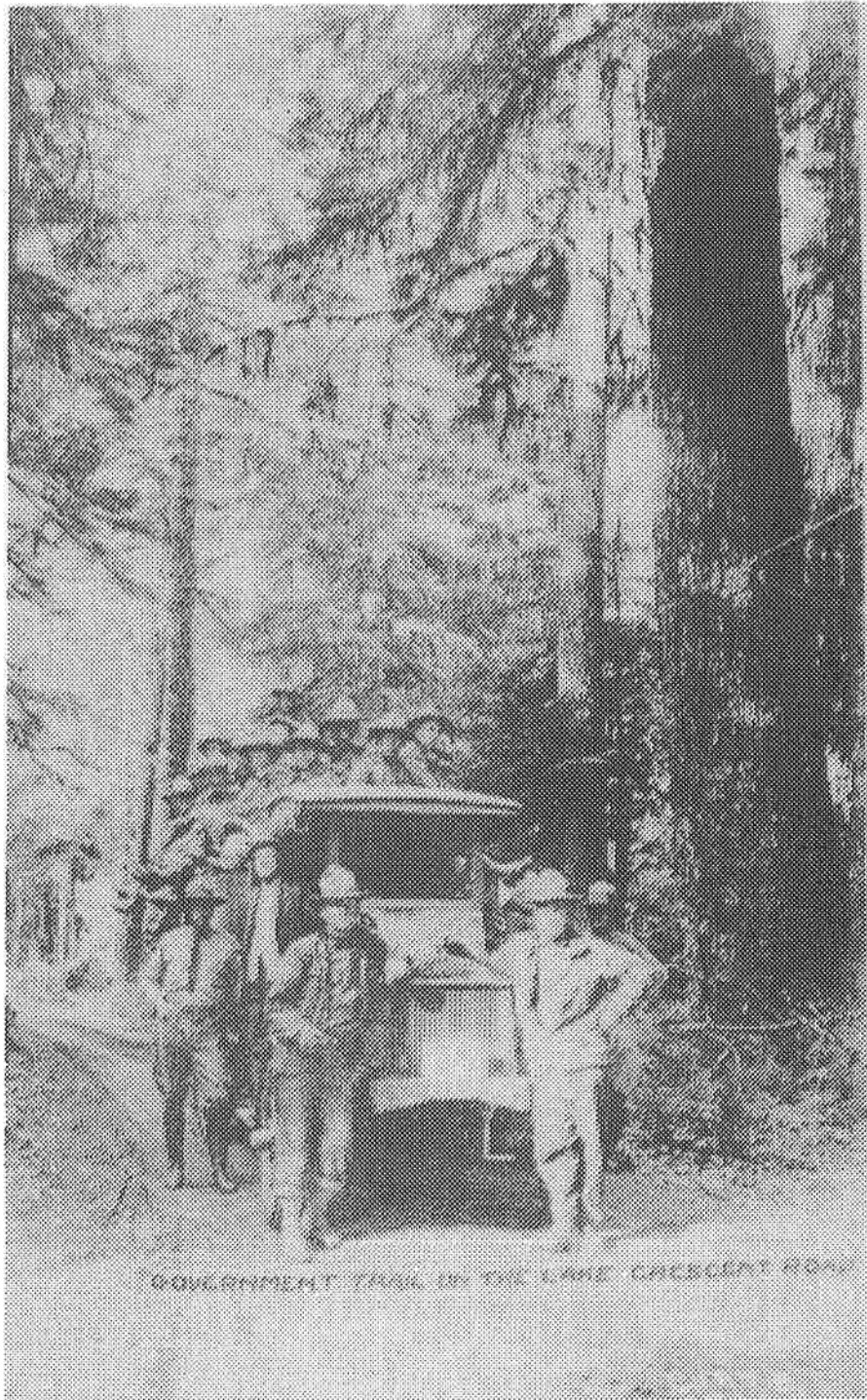
SPD truck used to haul men and equipment to construction work.
