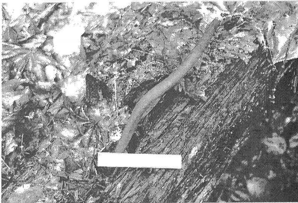
Photo W4-13 Trestle timber with drift pin, segment 5
