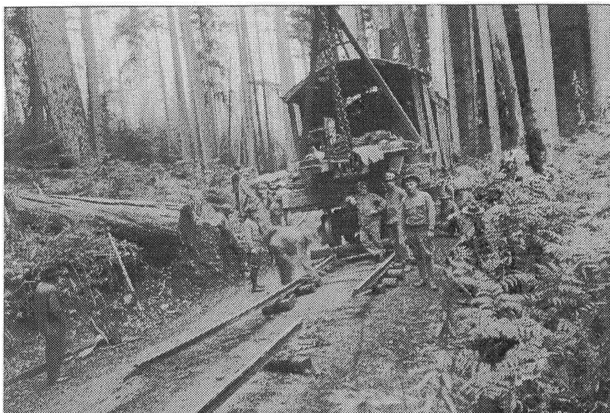
Steel gang laying rail with track-laying machine #38416
