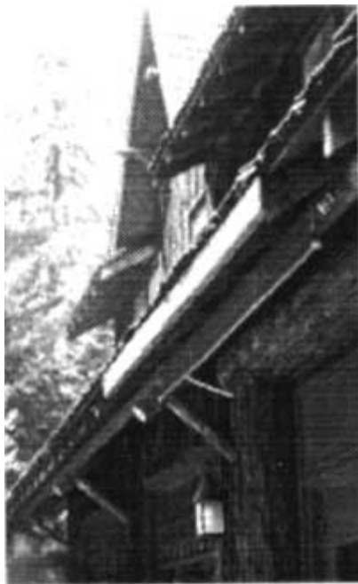
Fascia board for gutter.
