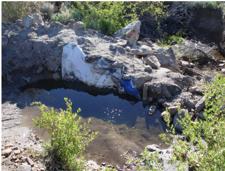
Figure 21. Looking downstream at pool constructed just downstream of City of Rocks road on Circle Creek.
