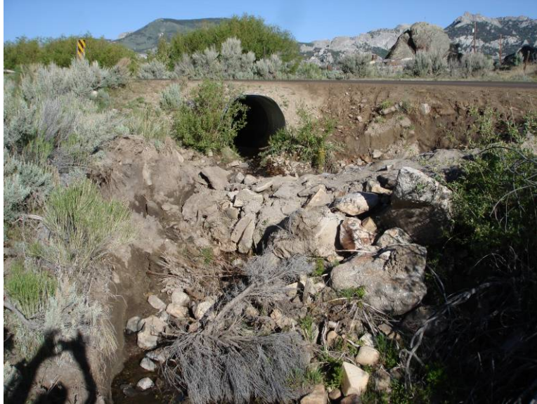
Figure 22. Looking upstream at pool constructed just downstream of City of Rocks road on Circle Creek.
