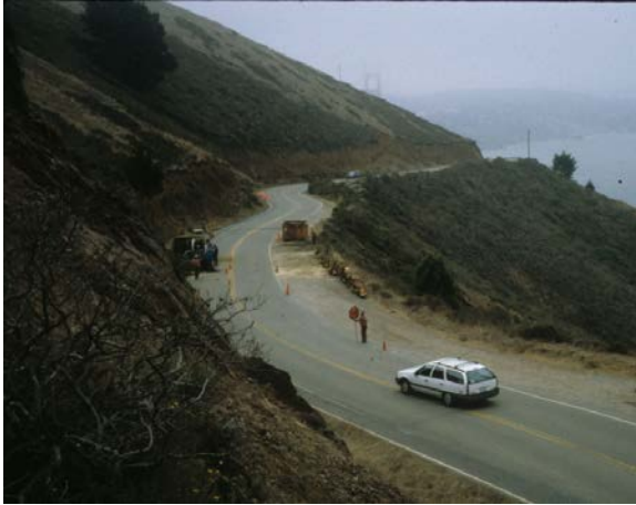
Figure 4 – Traffic control on Conzelman Road.
