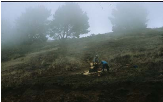
Figure 5 – MCC crew members flush cutting tree trunks on Slacker Ridge.
