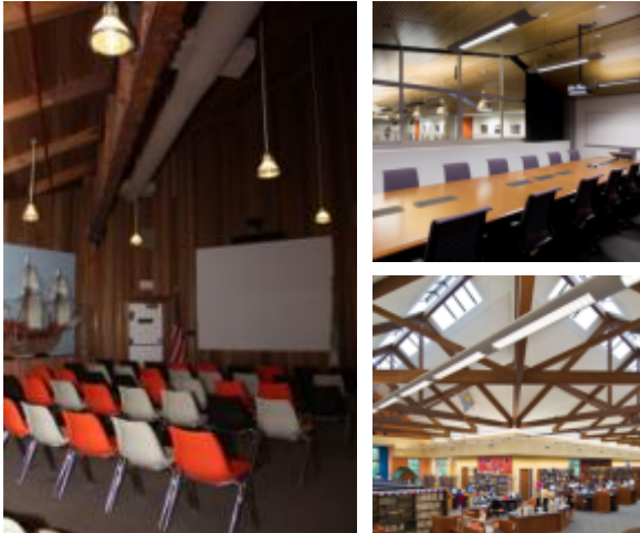
Figure 15: BVVC A/V room (left), Finelite indirect / direct A/V lighting (top right), Finelite indirect / direct lighting (bottom right).
