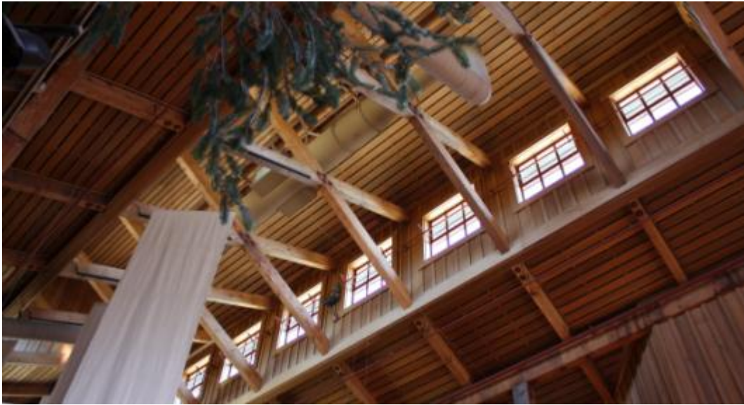
Figure 1: The interior ceiling of the BVVC and BVVC gable.
