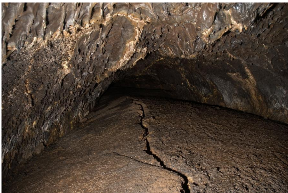
Figure 7. Contraction cracks in Catacombs Cave.
