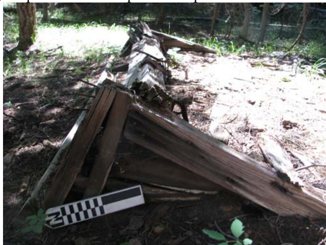
Figure 11: Photograph 07-14-2009-06. Side view of wooden structure (IF-CRLA-2009-22).
