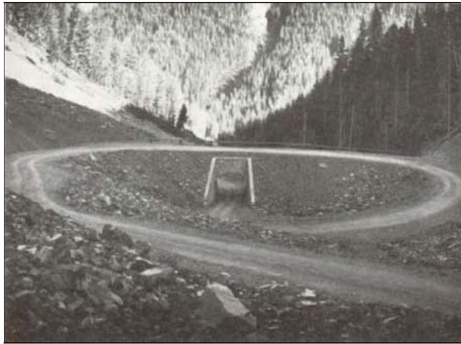
Fig. 6. The construction of the Cody Road with its Spiral Bridge depicted the early emphasis in park road construction. Engineering was of primary importance, aesthetics were secondary. ( National Archives, Record Group 70, n.d. )
