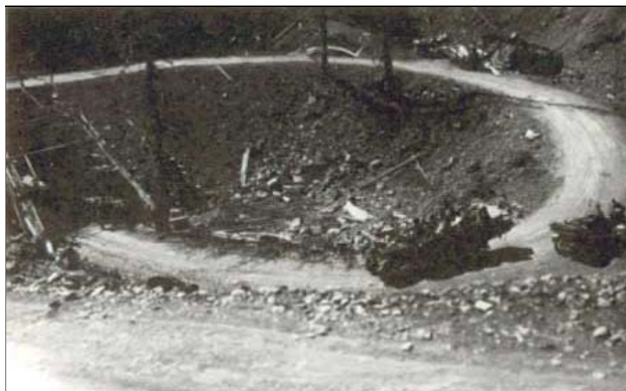
Fig. 5. At Yellowstone, the construction of the Spiral Bridge at "S" Hill over Sylvan
