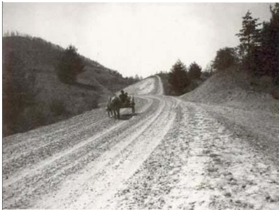
Fig. 21. Glimpses of Appalachian culture were visible along the parkway. This photograph of an ox cart trundling along the road was taken near Bluff's Park in April 1938. The contrast between the technically advanced ongoing construction work and the primitive local conditions was sharp. ( National Archives, Record Group 79, Rinehart Photo )
