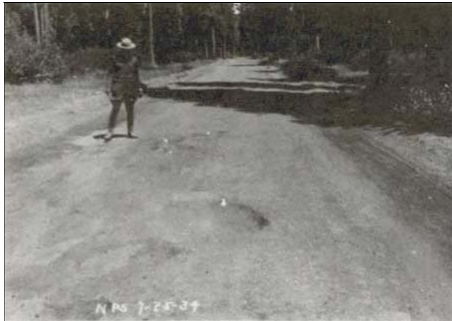
Fig. 7. During the 1920s the road system at Crater Lake had no surface, and the pumice gravel caused maintenance problems, such as this pothole. This photograph was taken of the south entrance road. ( National Archives, Record Group 70 )
