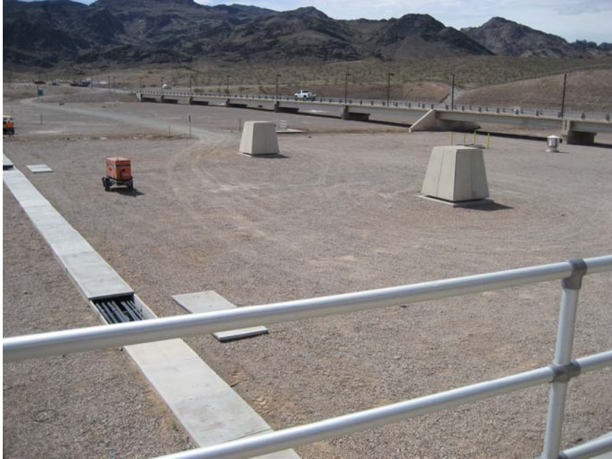
Fig. 34: Site above the underground clear-well storage tank at the SNWA pumping station.
