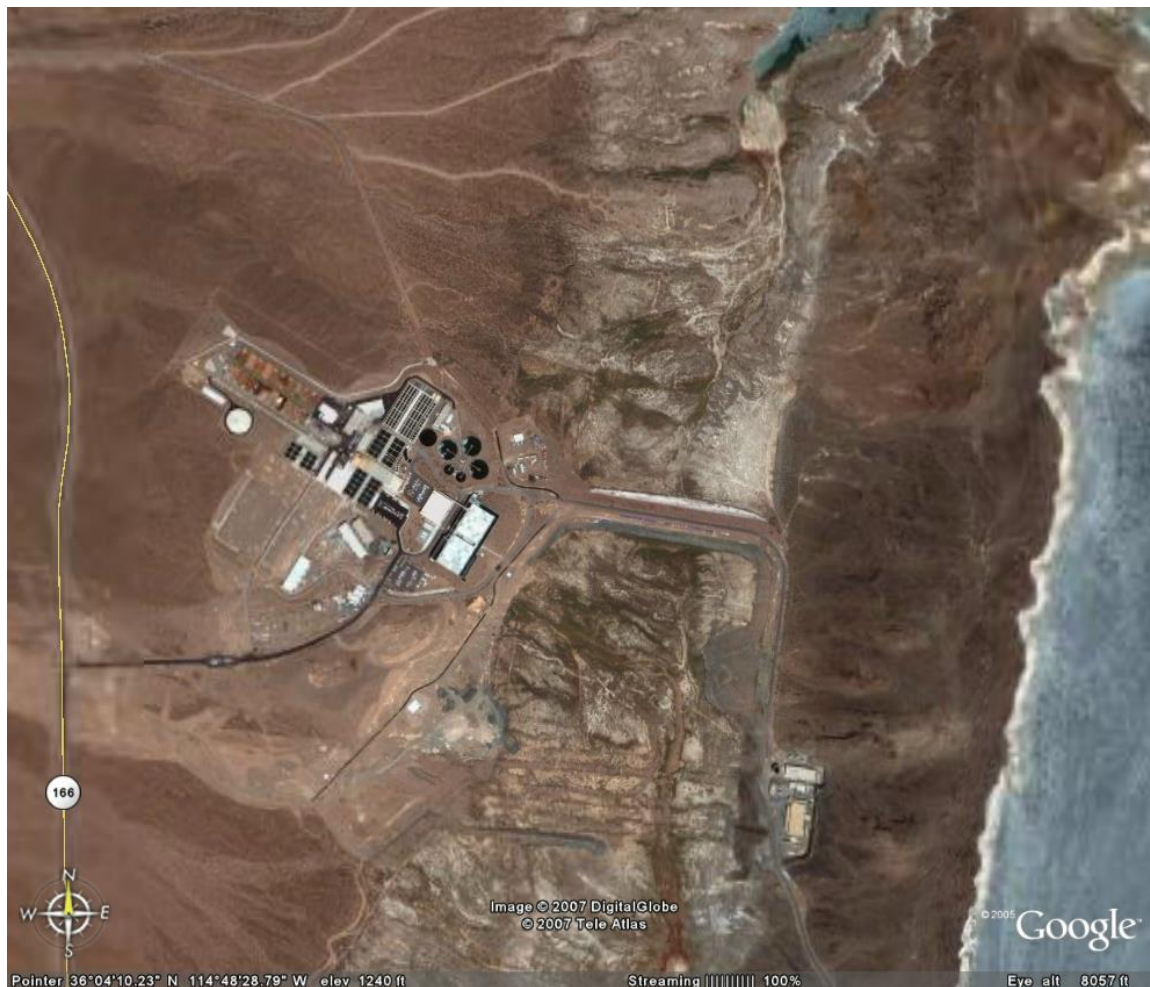
Fig. 29: SNWA pumping station; the western shore of Lake Mead is on the right.
