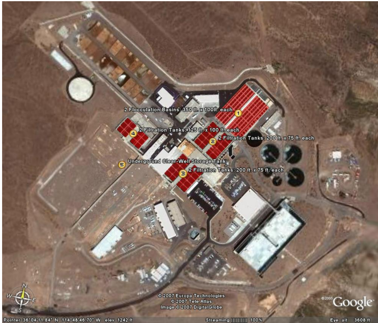
Fig. 31: Locations of potential photovoltaic sites at the SNWA pumping station.
