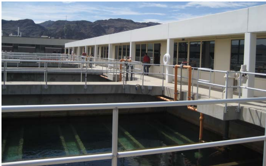
Fig. 33: Filtration tanks at the SNWA pumping station.
