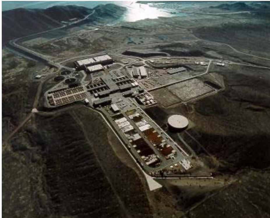
Fig. 30: Aerial view of SNWA pumping station; the shot is from the west looking east.
