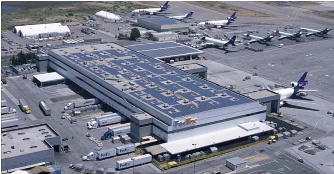
Fig. 39: The FedEx Oakland International Airport hub.
