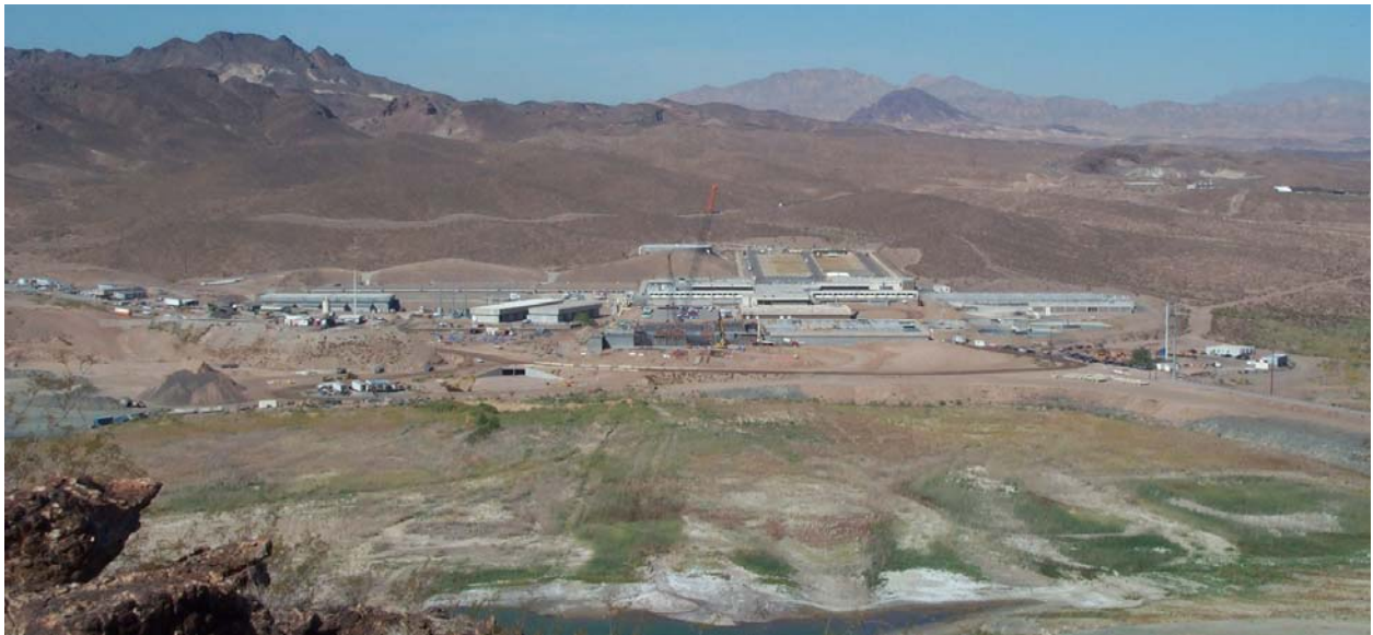
Fig. 36: Aerial view of SNWA pumping station, looking to the west.
