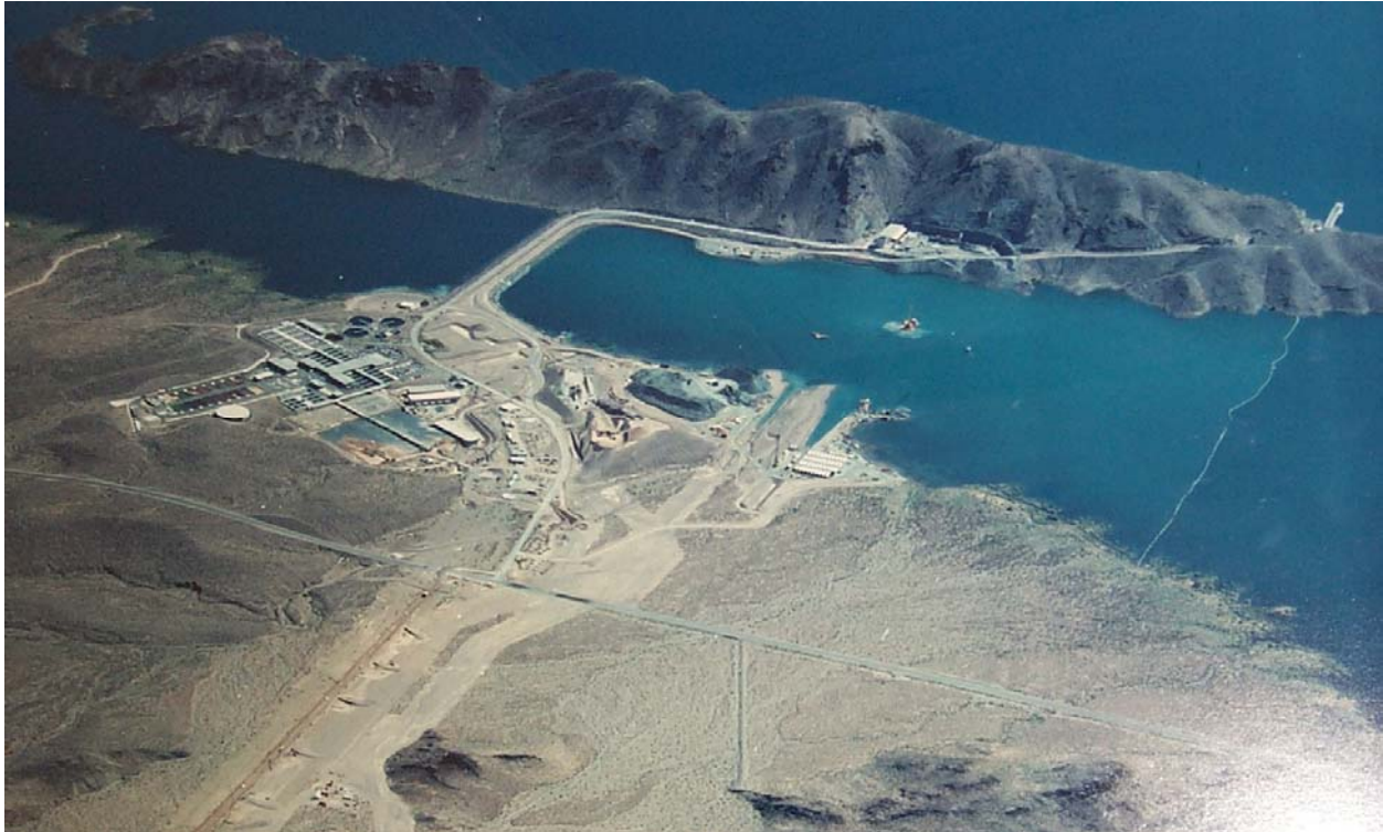
Fig. 35: Aerial view of SNWA pumping station, looking to the east.
