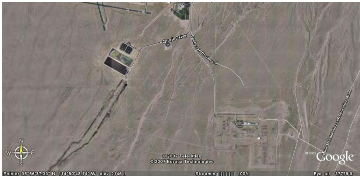
Fig. 28: SNWA treatment plant and nearby power substation.
