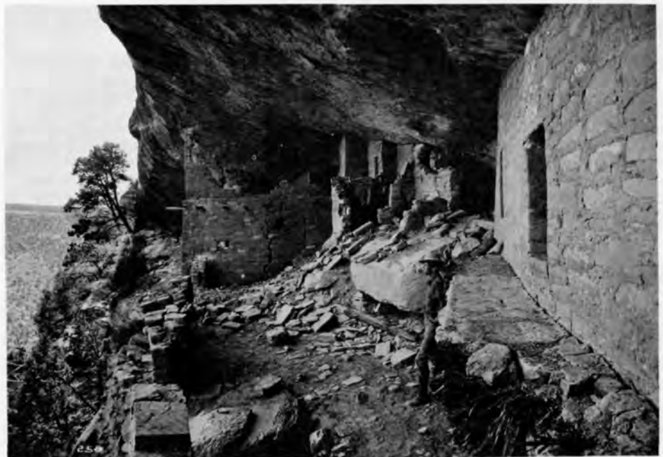
Balcony House before repairs. Mesa Verde NP, Colo. Photo by Nusbaum, 1910.
