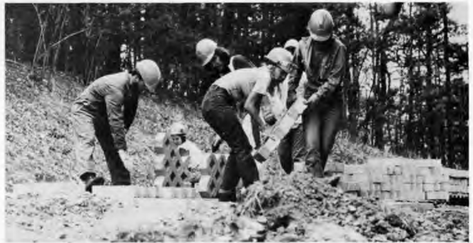
At the North Carolina end of the Blue Ridge Parkway, YACCers helped to lay prefab turf blocks, which are installed next to the roadbed.
