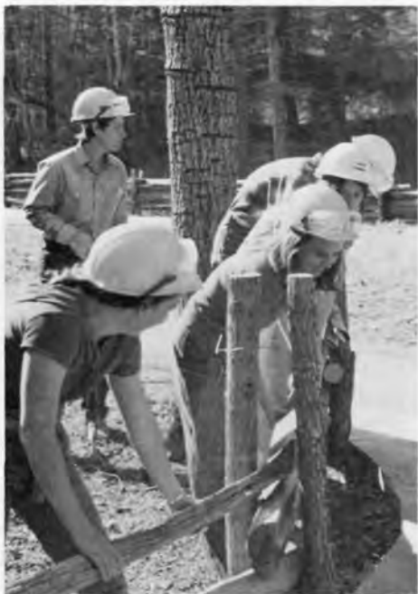
James River YACC crew repairing fences at the entrance to the Otter Creek Restaurant and Craft Shop, Blue Ridge Parkway, N.C.-Va.
