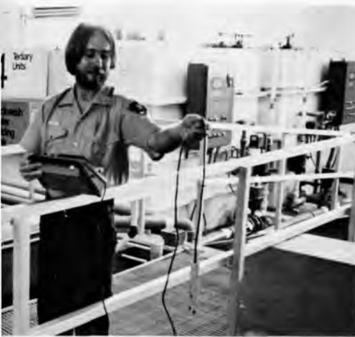
Wastewater treatment plant operator drops a probe into a tank to measure oxygen levels in the treated waste water.
