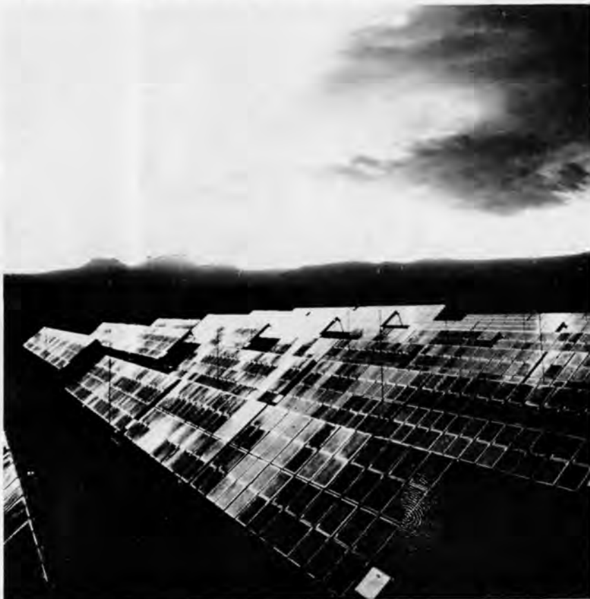
Solar collector panels atop Natural Bridges' new solar photovoltaic system help provide all of the electricity needs of the national monument.
