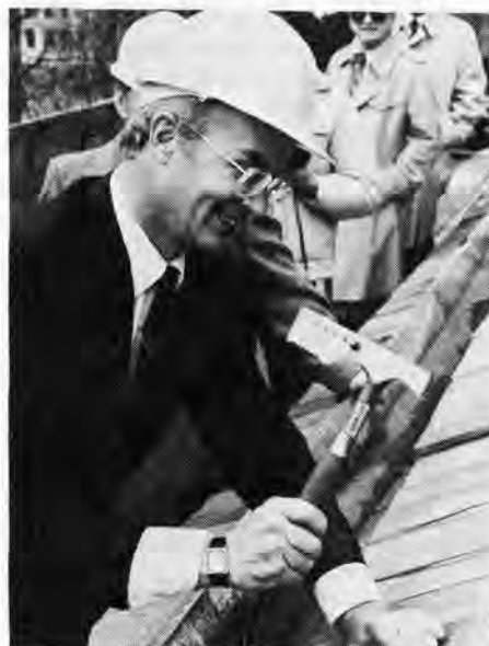
Secretary Watt nails a cedar shingle to the roof of Congress Hall.
