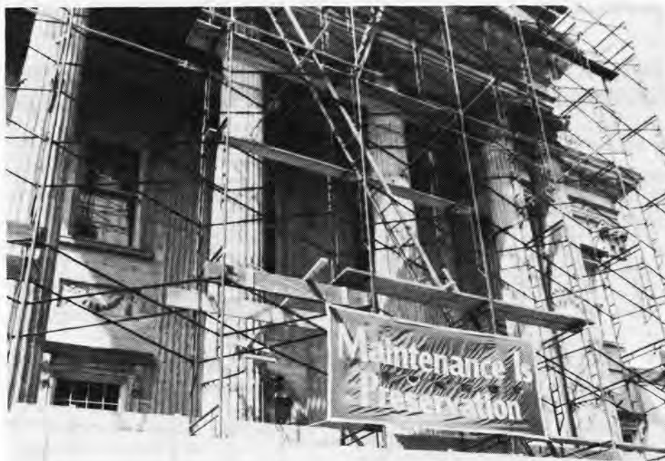
The staff of Independence NHP put up this banner to tell the public of the current restoration work on the historic First Bank of the United States.
