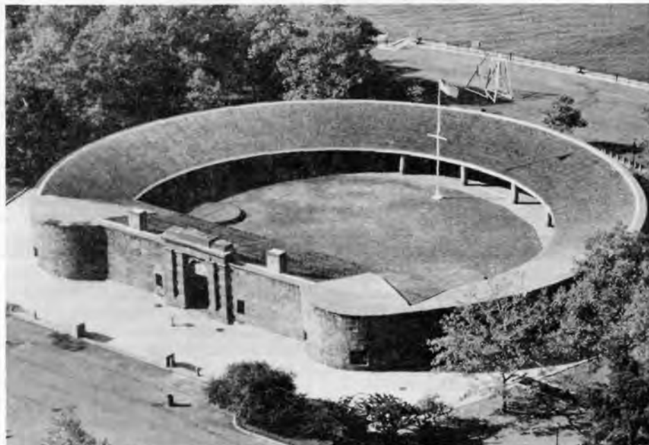
Castle Clinton prior to restoration
