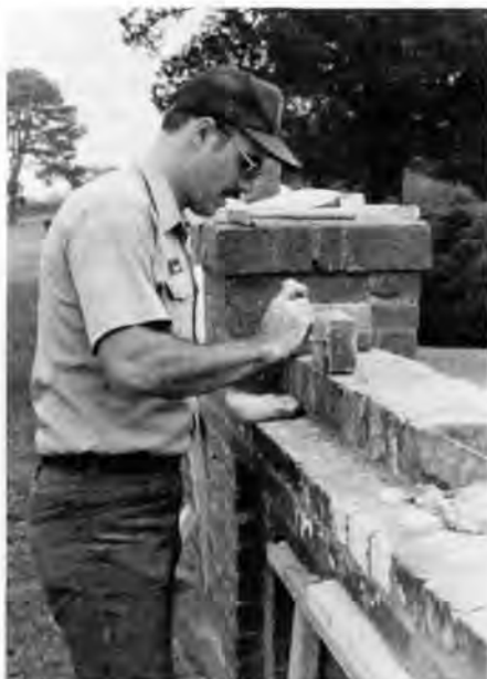
William Bonsall (Independence) in the process of tack-pointing (forcing mortar into the brick for a water-tight seal). Photo by A. Myers
