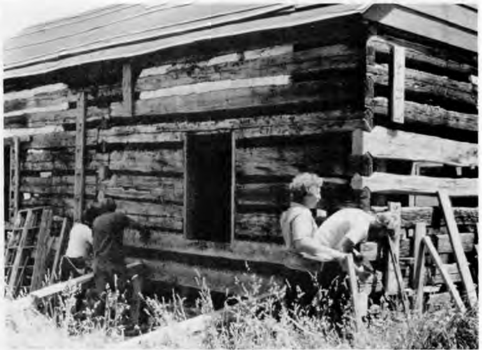
Trainees from the Williamsport Preservation Training Center replace a log on the Slave Quarters at Hampton NHS, Towson, MD. Photo by Emogene Bevitt.
