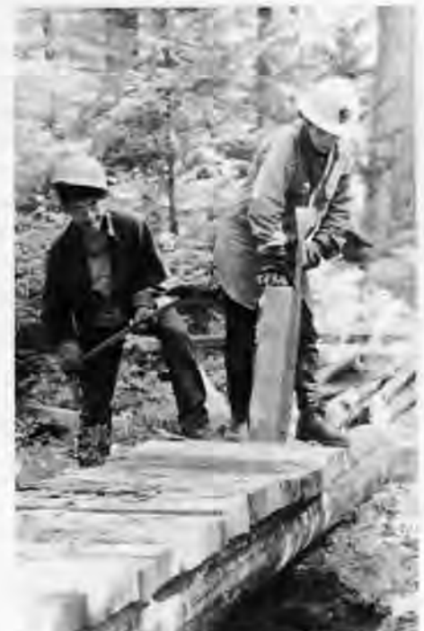
Building puncheon in North Cascades
