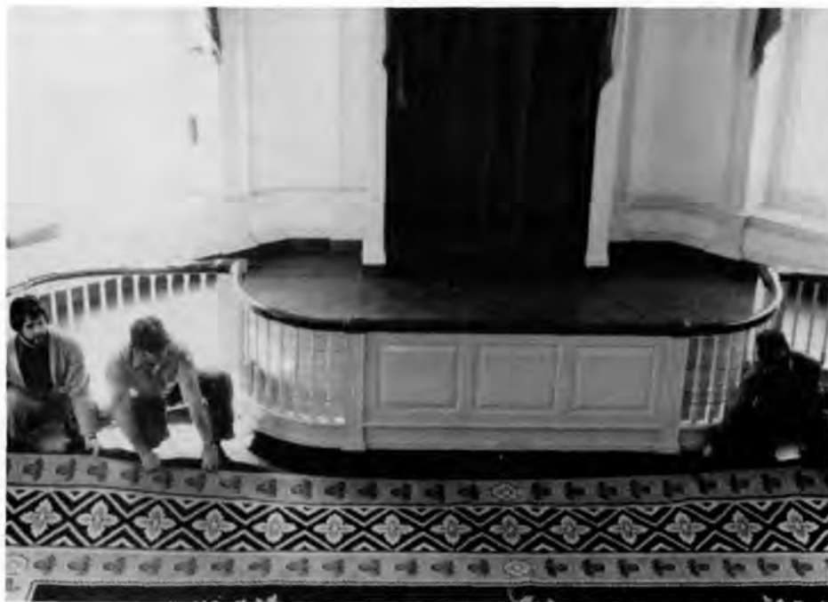
Installation of new carpet, Congress Hall Senate Chamber (photo courtesy of Independence NHP).
