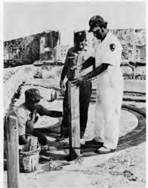
Mason Efraín Santiago, maintenance supervisor Rosendo Figueroa and mason's helper Antonio Trevino shape ausubo (bullet wood) to fit a hole at the end of the cannon track. Rot and termite resistant ausubo saved from old buildings is the same used by the early Spanish fort builders so the maintenance is historically correct and safetywise so visitors cannot trip in the hole.
