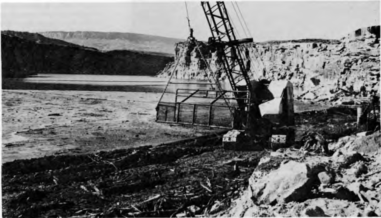
OIL SOAKED DEBRIS IS REMOVED FROM LAKE POWELL by a Texas-New Mexico Pipeline Company crane basket. Debris is backed up by the log boom at the San Juan arm of the lake. The crane was brought to the site aboard the NPS 52-foot landing craft, a 200 mile round trip from Halls Crossing.
