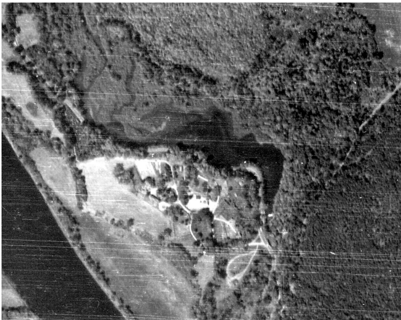
Figure 16. Aerial photograph from 1952 showing the Blow-Me-Down Farm. The Blow-Me-Down pond is at image center and the Connecticut River is at image left. (SAGA files)
