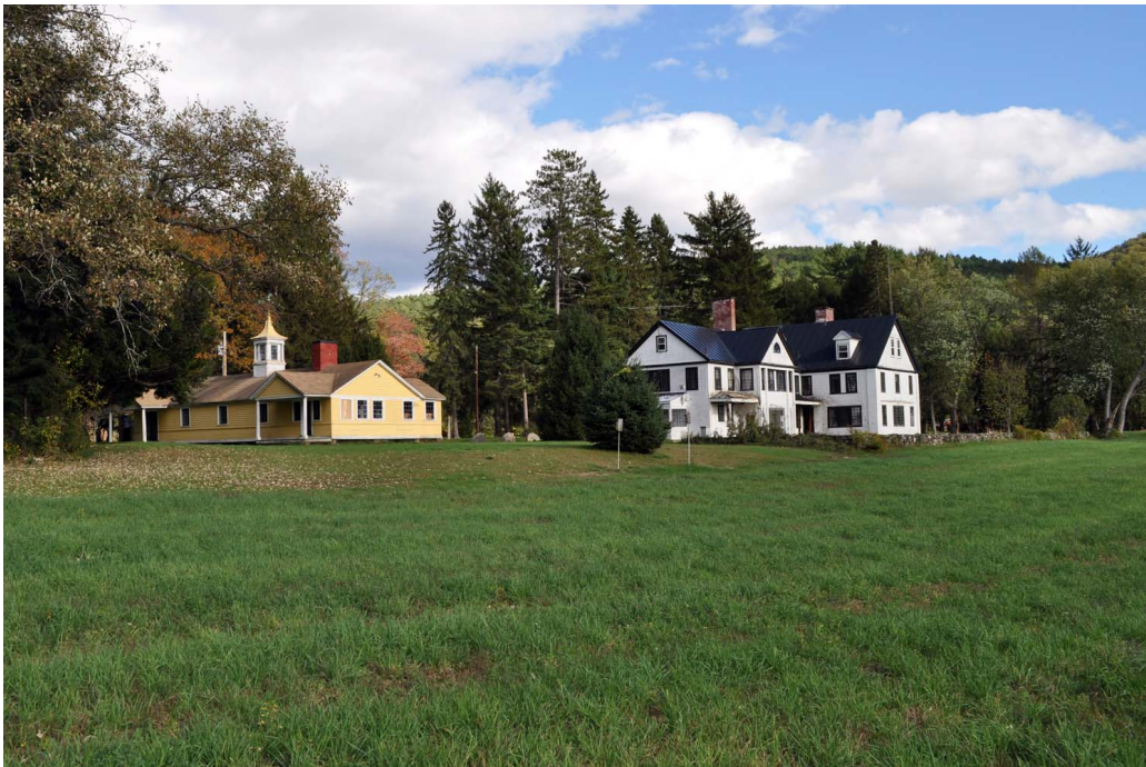
Figure 25. View looking east at the 1927-1929 dance hall (image left) and the 1888/1927 casino. The viewpoint of this photograph is similar to Figure 15. (OCLP, #DSC-0753, June 2013)
