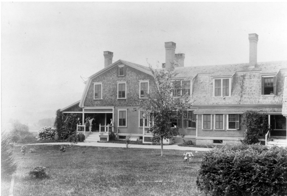
Figure 8. View looking west at the east side of the Blow-Me-Down cottage, before 1892. Trees and shrubs dot the lawns/meadows, and vines shade the porches. Note the gravel driveway along the building. (SAGA, 3065y-tif633640014133100134)
