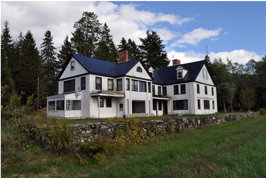
Figure 29. View looking east at the L-shaped stone wall on the south side of the casino. The top of the flagpole that stands in the middle of the driveway turnaround on the east side of the casino is visible at image right. (OCLP, #DSC-0756, October 2012)
