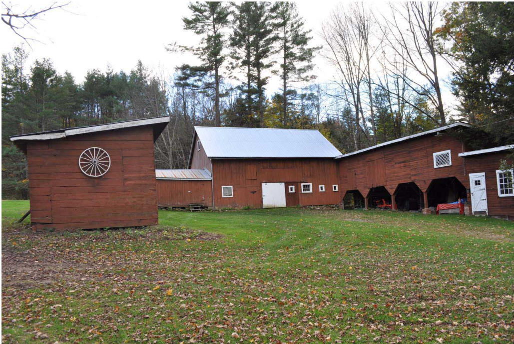
Figure 25. View looking south at the u-shaped barn complex, which houses maintenance equipment. (OCLP, October 2012)
