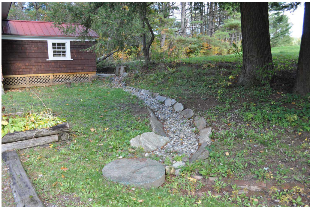
Figure 27. View looking north at stone and brick drainage swales that direct water to the east of the farmhouse into a covered culvert. (OCLP, October 2012)
