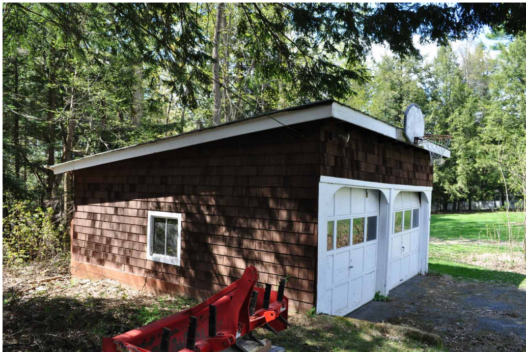
Figure 26. View looking northwest at the two-car garage used by the Saint-Gaudens caretaker (OCLP, May 2013)
