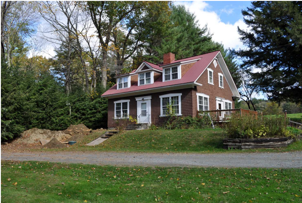
Figure 23. View looking northeast at the Saint-Gaudens Farm house with the driveway and front steps in the foreground. Concrete steps lead to the west facing door. (OCLP, October 2012)
