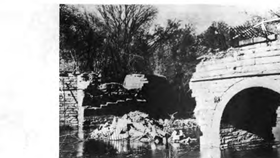
(Above) the collapsed Catoctin Creek Aqueduct, and the new Bailey Bridge, C&O Canal NHP, Md., D.C., Va.
