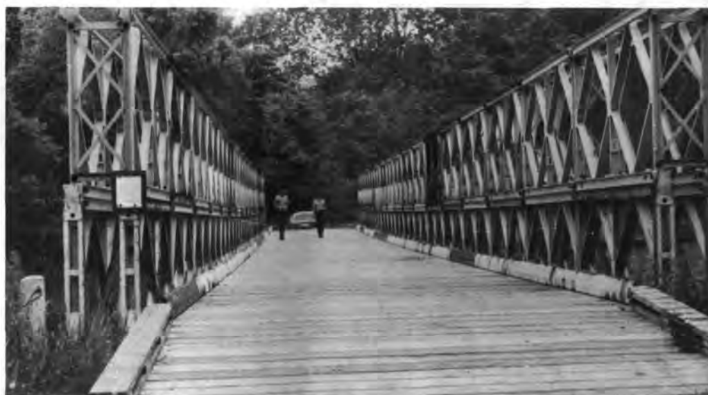
(Above) the collapsed Catoctin Creek Aqueduct, and the new Bailey Bridge, C&O Canal NHP, Md., D.C., Va.
