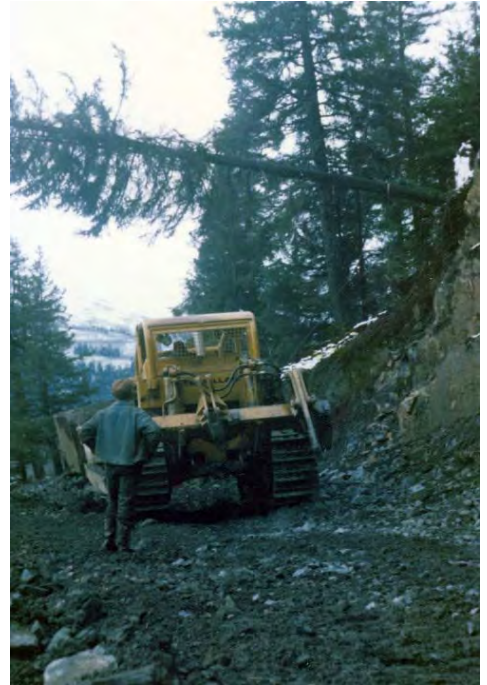
Building Exit Glacier Road. Photo: K.L. Freeman, Cooper Landing, Alaska, 1974.
