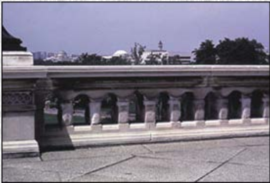
The marble balustrade on the west side of the Capitol building shows damage from acid rain dissolving the mineral calcite.
