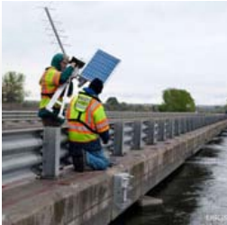
Photo: USGS crews install a rapid deployment streamgage on the Boise River near Parma, Idaho, in 2012. Credit: Tim Merrick, USGS.
