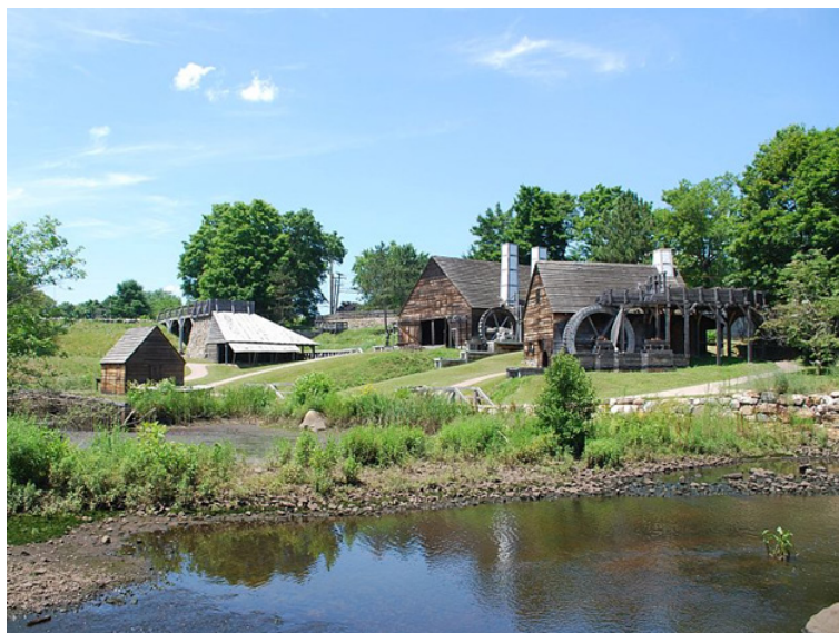
The iron works buildings and restored Turning Basin. Bill Gawley photo.
