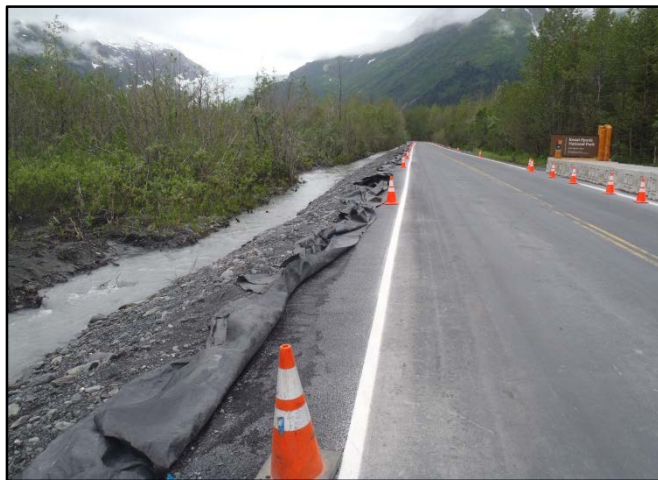
Figure 4: Road construction along Herman Leirer Road
